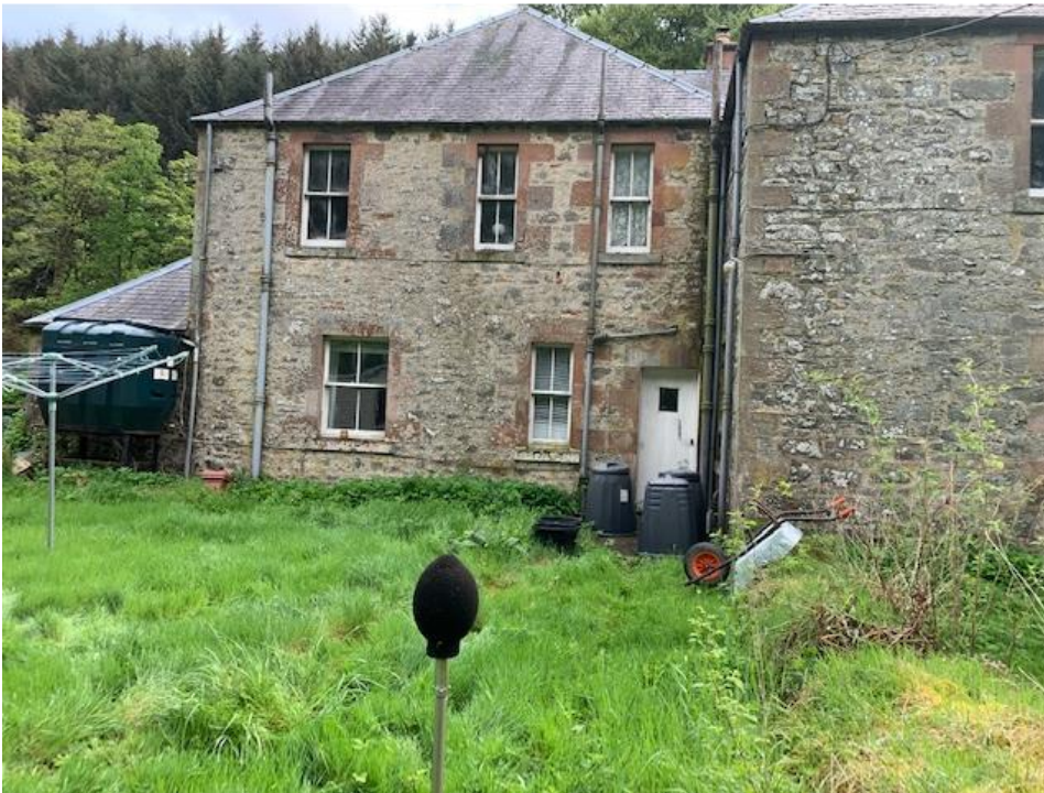
Figure C11 View of the monitoring location at Hyndlee looking east
