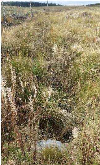
View upstream (SW) showing culvert pipe and narrow overgrown channel
